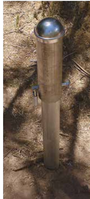
Riser from a temporary groundwater monitoring well in Granite Camp. The wells will be removed when staff have collected adequate data on groundwater levels.
