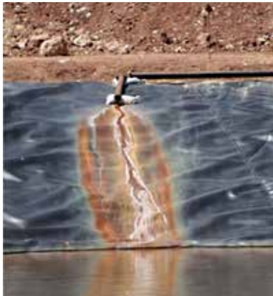
Sump water catchment pond at Pinenut Mine. Photo: Taylor McKinnon
