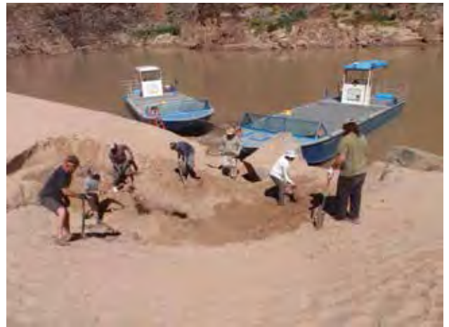
Crews filled in large ravine near pull in area at Bridge Canyon City camp with nearby material from cut bank to facilitate campsite set up and overall safety. photo: NPS photo.
