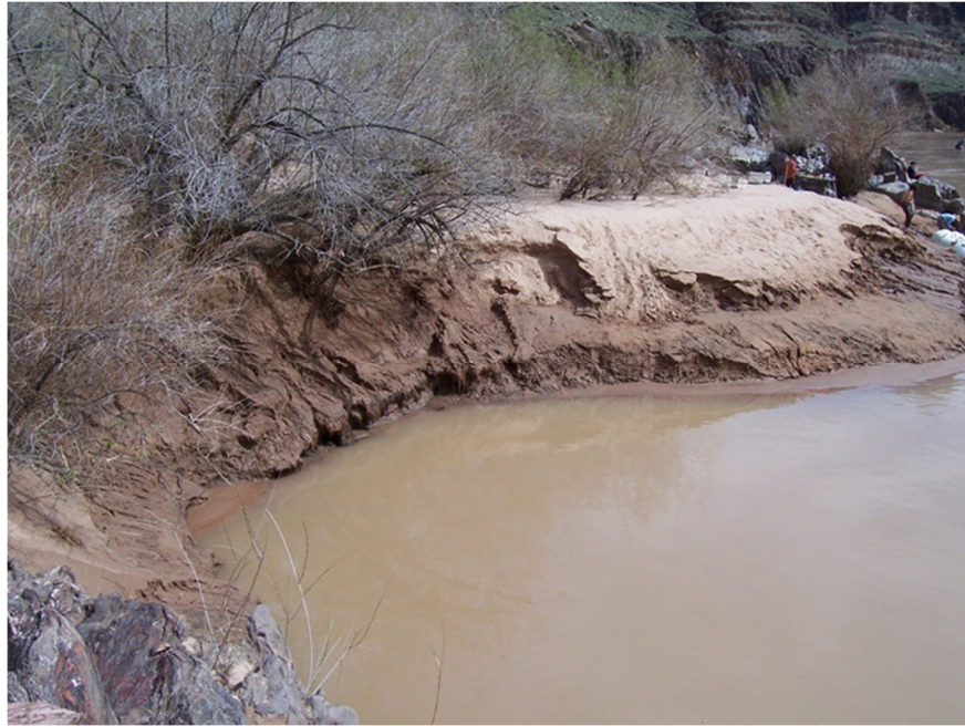
Figure 23. Beach being undermined by water drainage after HFE due to quick downramp. Bass Camp, RM 109.1 R, March 14, 2008.
